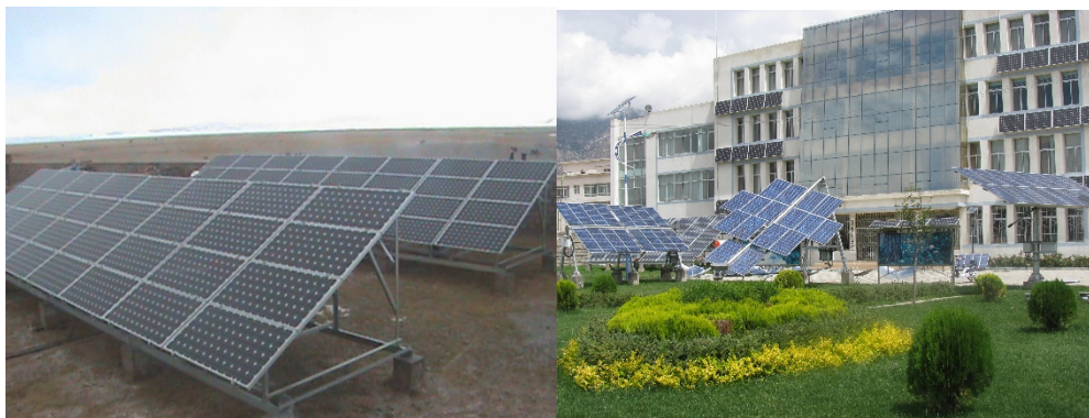
Fig. 4 Application of independent photovoltaic power station in Tibet
