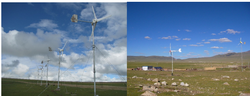
Fig. 5 Application of wind solar complementary power station in Tibet
