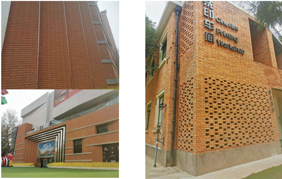
Fig. 9 Shaped wall with red brick as base material (top left and right) Red brick + stainless steel + perforated aluminium panels (bottom left) (Source: Image from the Internet)
