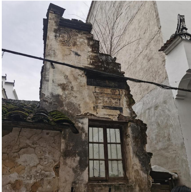
Figure 1: Current situation of some buildings in Tsinghua Town
