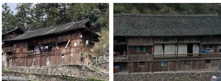
Figure 1. Selected stilt house test building
