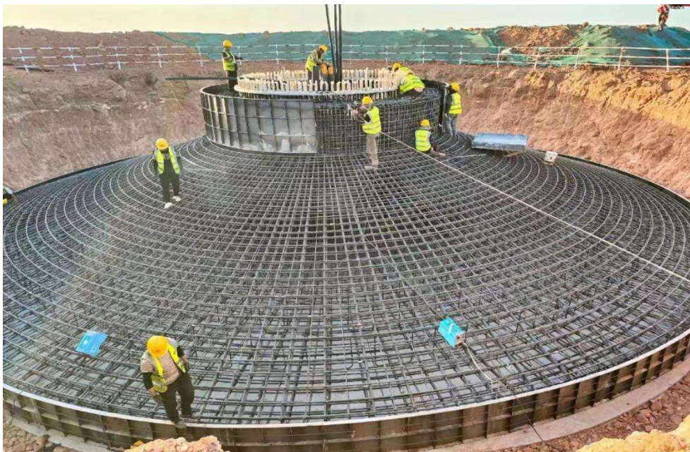
Fig.8 Fan foundation reinforcement layout
