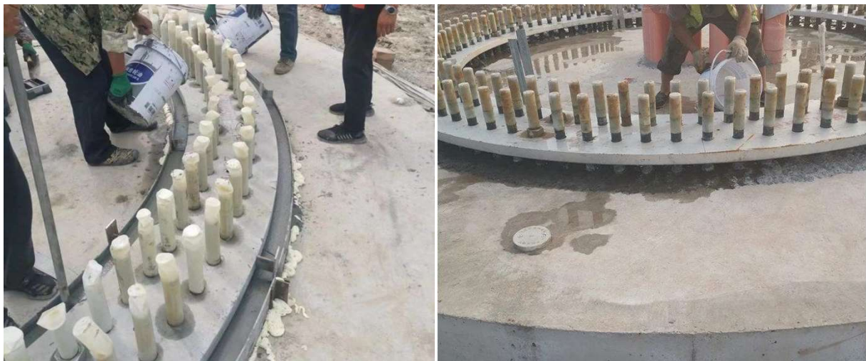
Fig.10 Grouting construction
