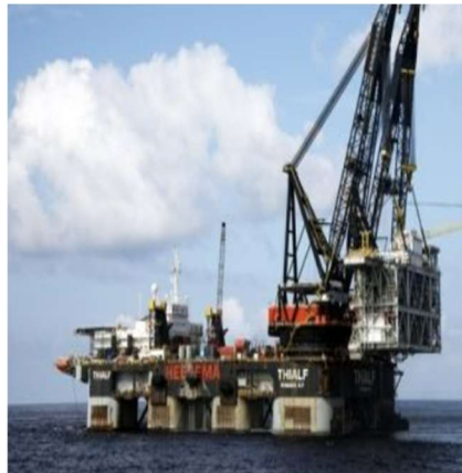
Figure 1. Thialf Semi-submersible Crane Vessel
