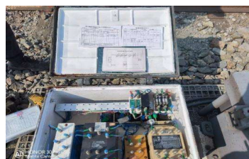
Figure 8. Internal diagram of power transmission box
