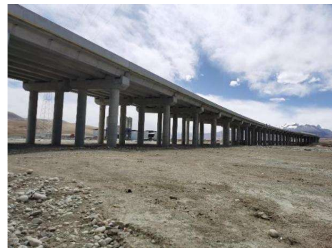
(b)The right elevation of the bridge
