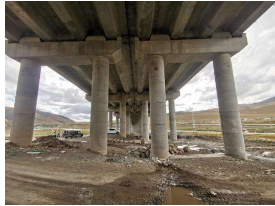
(d)Bottom view of bridge
