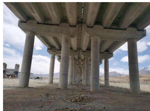
(d)Bottom view of bridge
