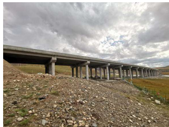
(b)The right elevation of the bridge
