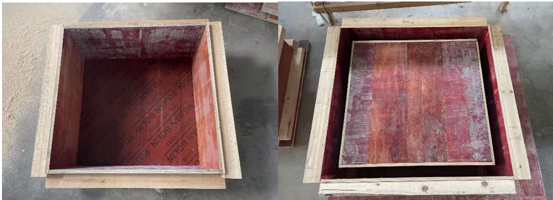
(a) Photographs of the Foundation Formwork (b) Photographs of the Excavation Formwork Figure 1. Fabrication of Wooden Formwork
