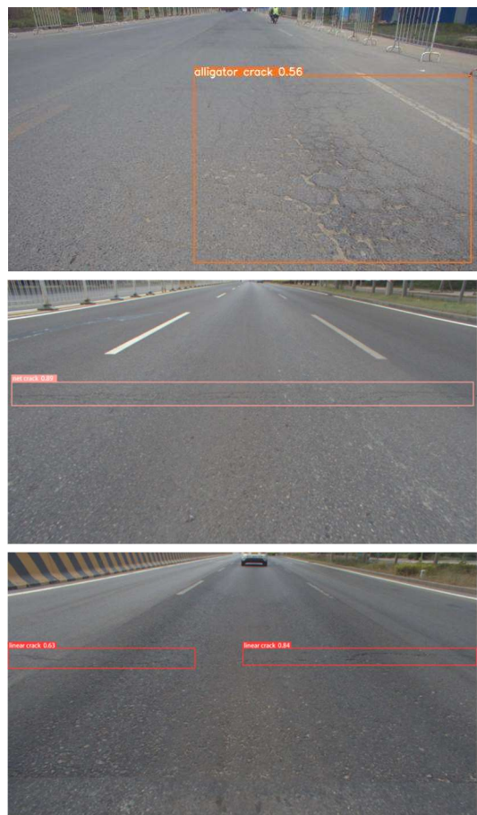
Figure 7. Detection results of road surface images
