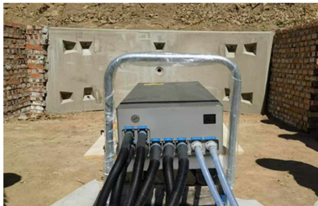
Fig. 1 Experimental site of continuous detection of voids behind segment based on impact echo method
