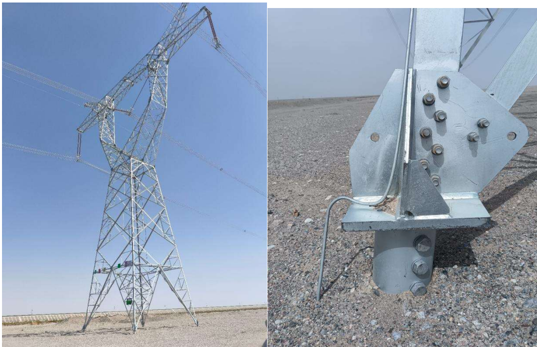
Figure 3. On-site Photo of Completed Helical Anchor Foundation Connection Node
