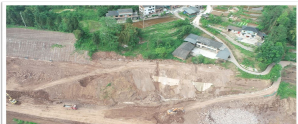
Figure 3. Photographs of slope construction during the pre-flood survey
