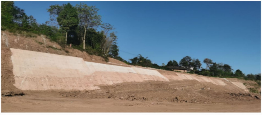
Figure 4. Photographs of slope construction during the post-flood survey
