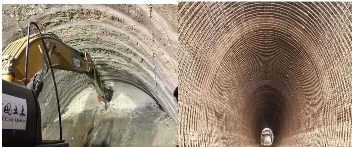
Fig.3 Steel mesh lining in Ganseta tunnel construction
