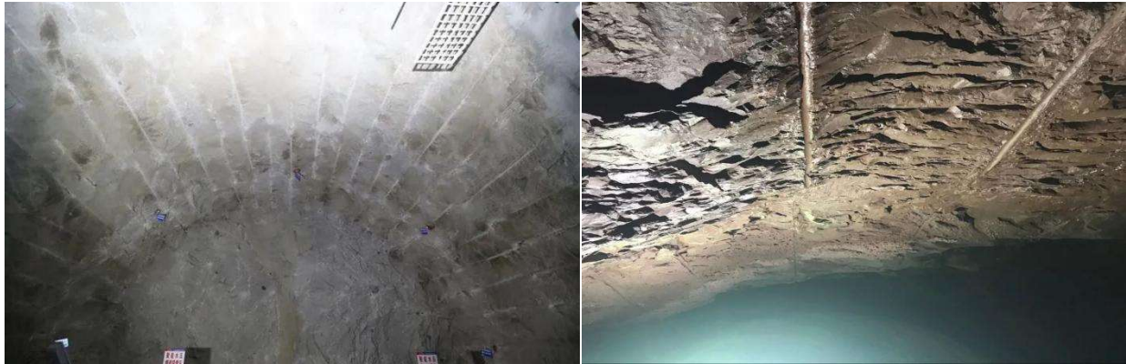
Fig.12 Smooth blasting effect of condenser water pressure
