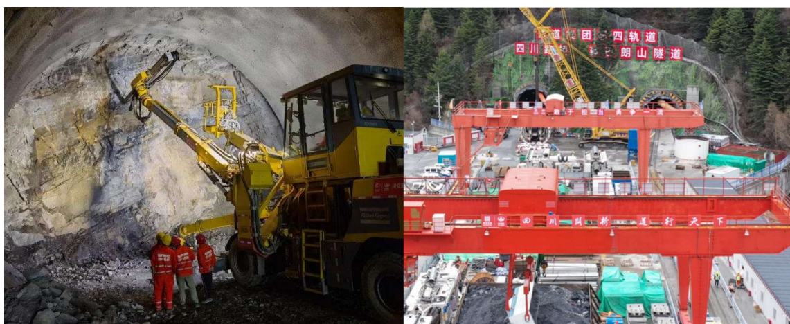
Fig.5 Construction of Yanjiang Expressway and Dusi Railway Tunnel
